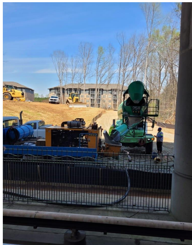
Concrete pouring for new platform
