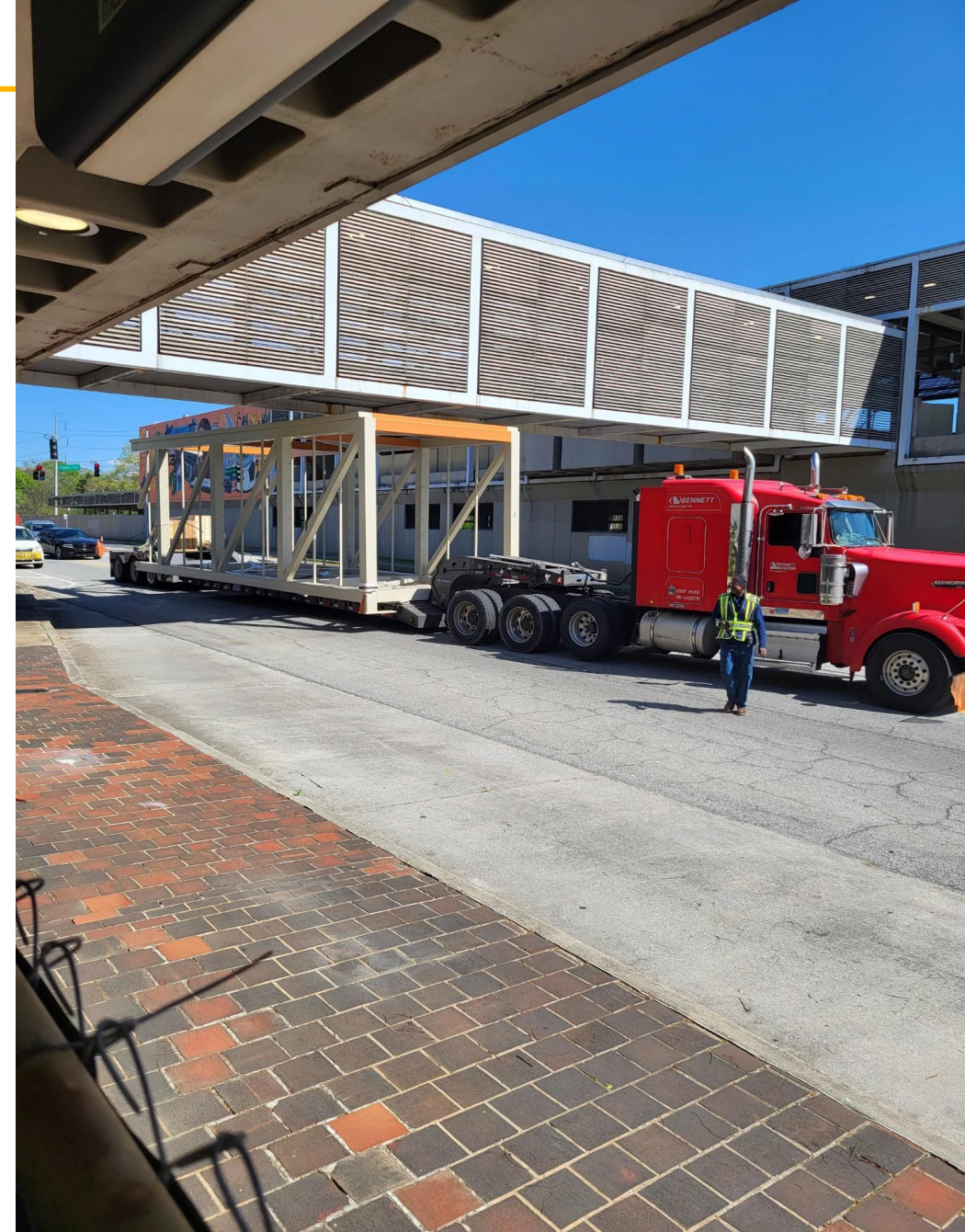
New bridge under the old bridge
